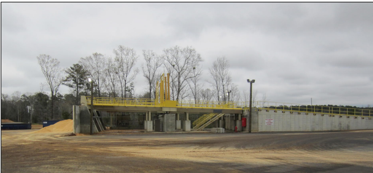
Figure 4-3 Elevation View of Back-on Style Truck Tipper with no Dumper Hopper or Dust Collection (Demopolis)
