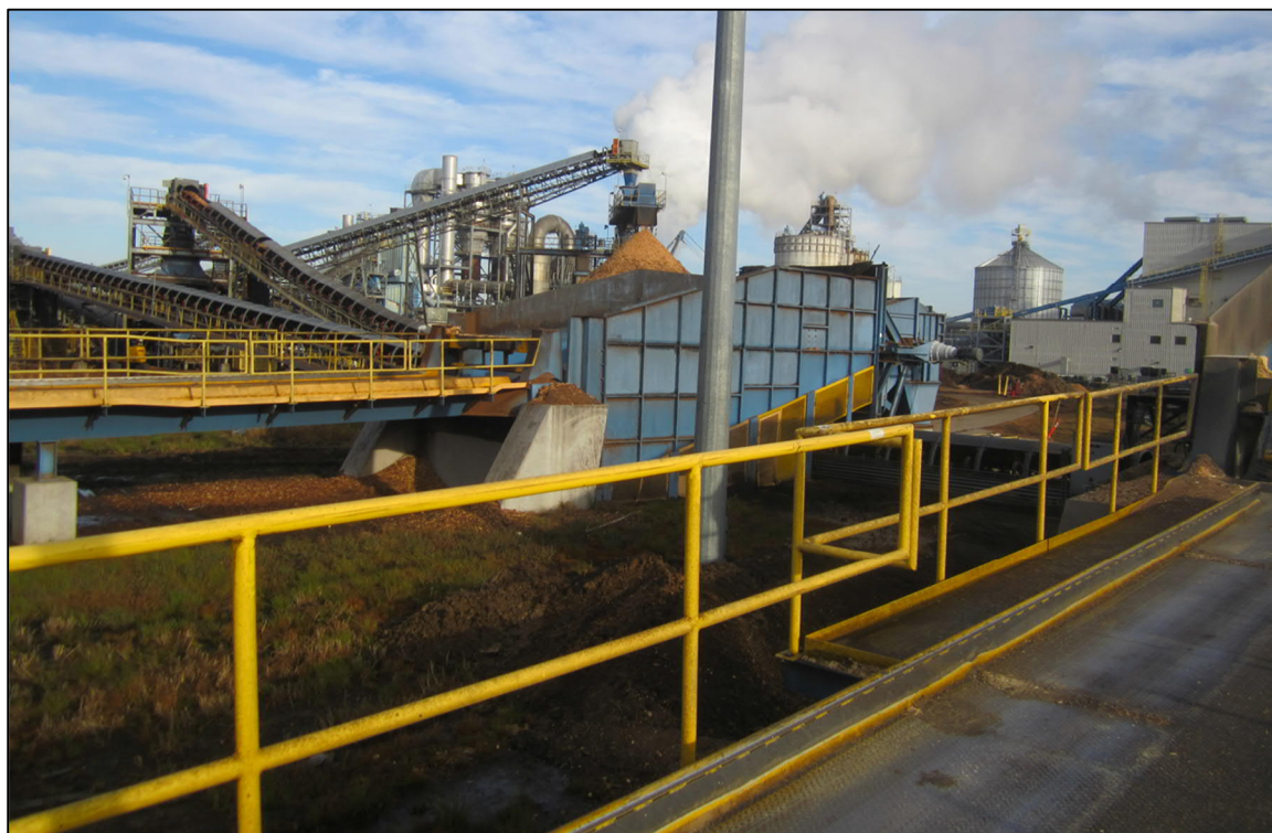
Figure 4-5 Elevation View of Back-on Style Truck Tipper with Near Grade Dumper Hopper (Drax Morehouse Facility)
