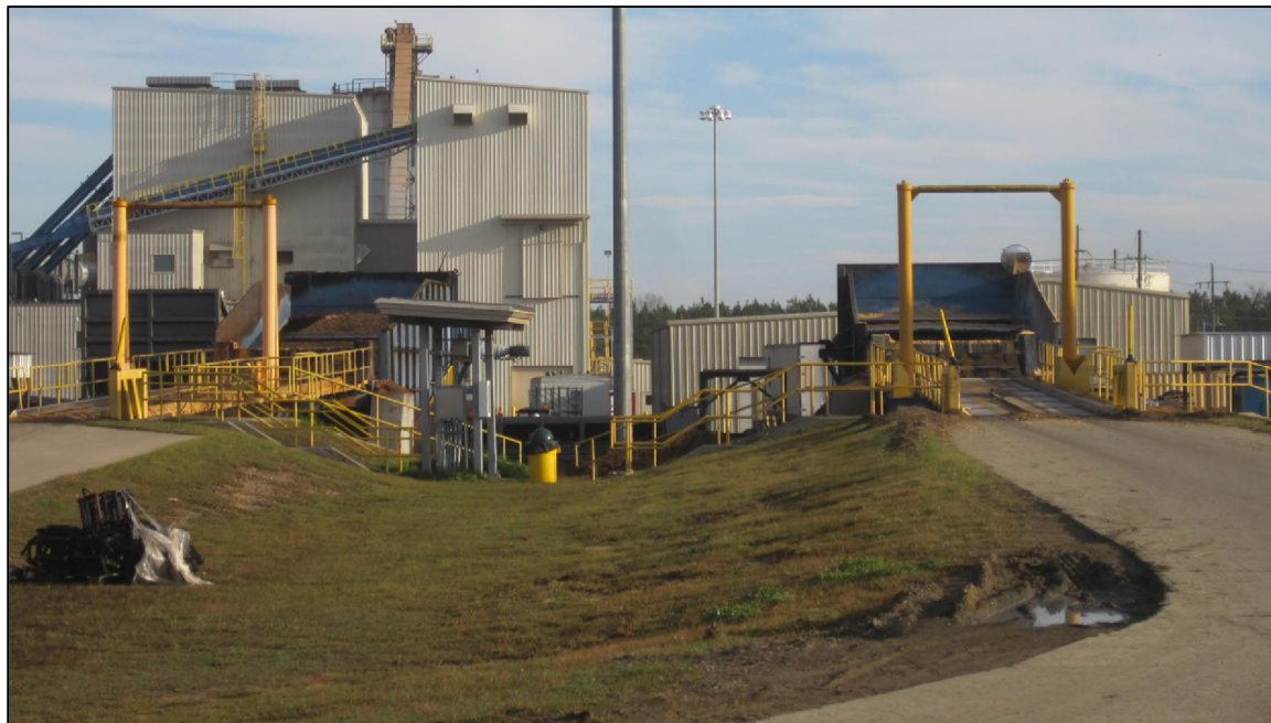
Figure 4-4 Back-on Style Truck Tipper with Near Grade Dumper Hopper (Drax Morehouse Facility)
